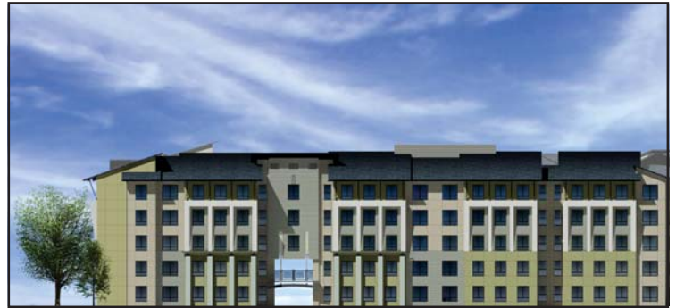
Design for Student Housing Project, Cal Poly San Luis Obispo Building 5 Neighborhood 3
